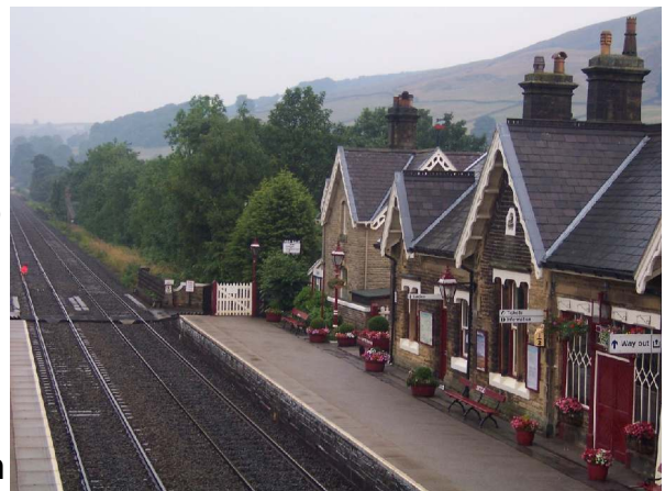
Settle Station as seen from the Station B&B
